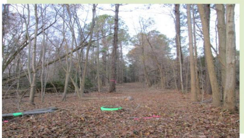
Cleared Right of Way over a Cross-Country Sewer Line
