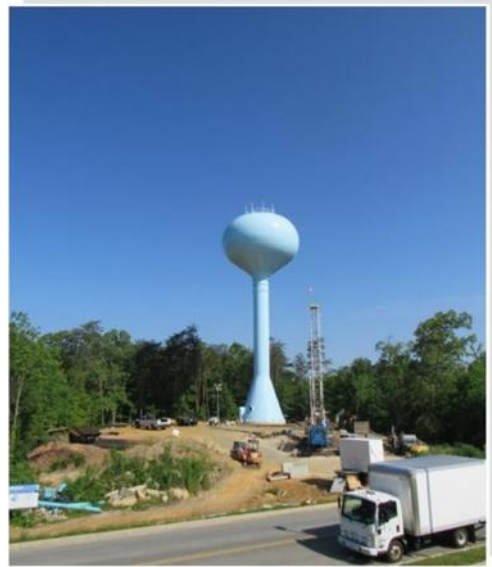
Charlotte Hall Tower Project: Well Drilling
