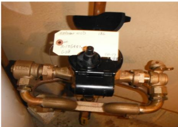
Automated Meter Reading (AMR) Project: New Indoor Residential Water Meter Installation
