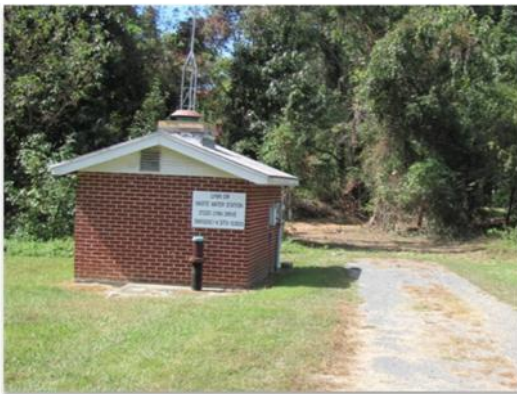
Lynn Drive WWPS & Forcemain Replacement: Station Before Replacement
