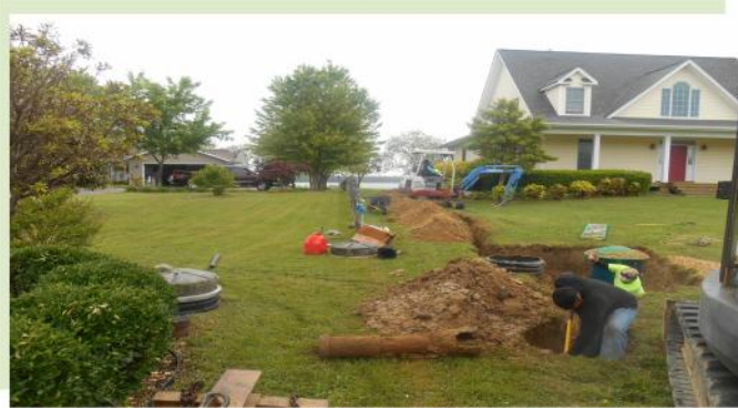
Contractors installing a replacement sewage grinder pump
