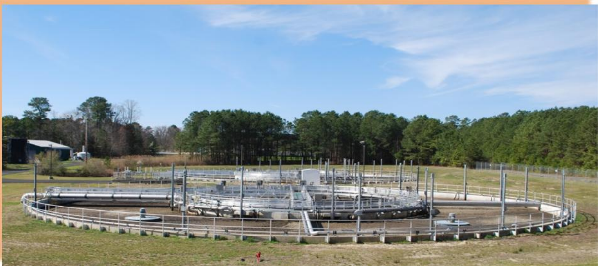
MTWRF ENR Upgrade Project: Completed Reactor Modification
