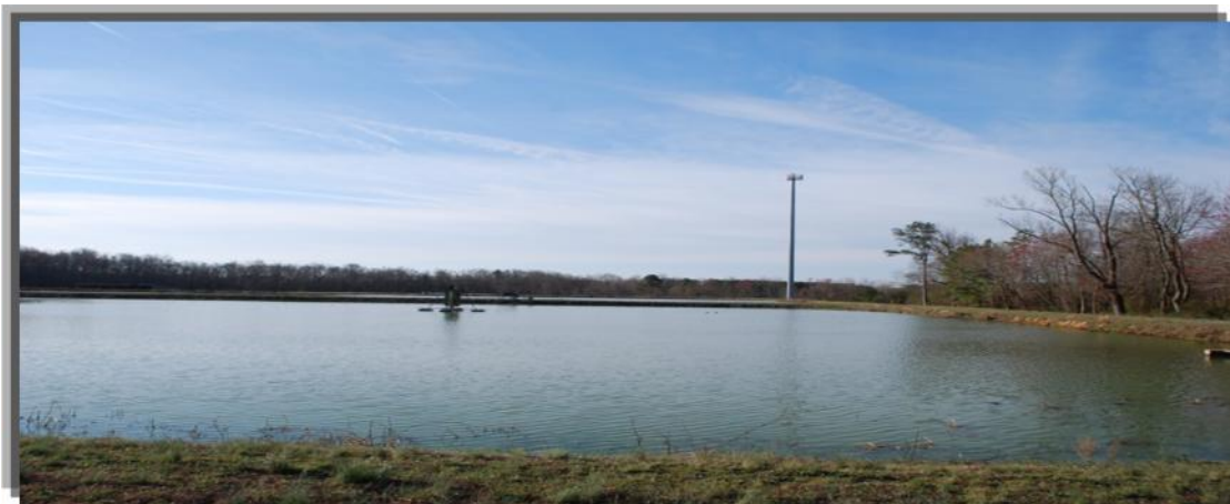
St. Clements Shores WWTP: Existing Lagoon
