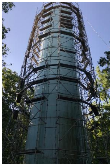
(Left Photo) Scaffolding set up at the Paw Paw Hollow in preparation for painting
