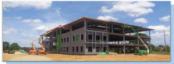
East Run Medical Building: Developer Funded Project Under Construction
