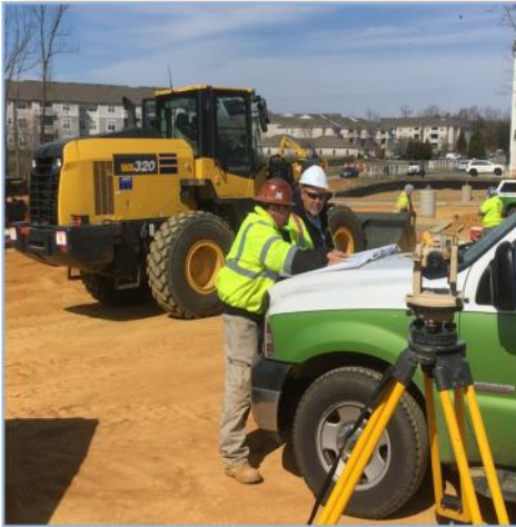
St. Mary’s Market Place: Developer Funded Project Under Construction
