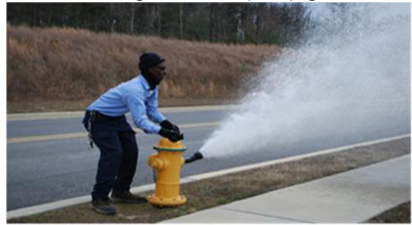
Water Operator Roy Person flushing a fire hydrant
