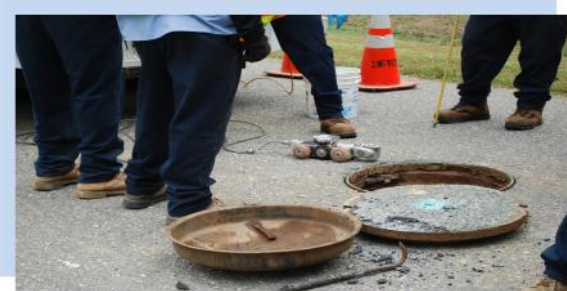
Sewer Rover Camera used to conduct inspections
