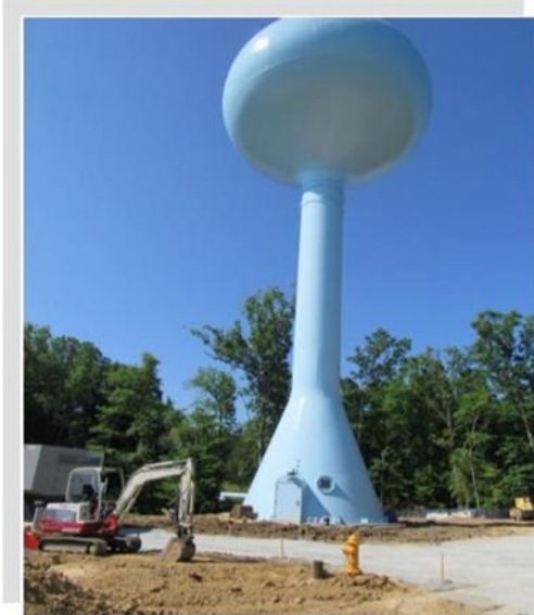
Hollywood Tower Project: Site Work
