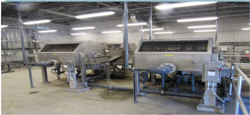
MTWRF ENR Upgrade Project: Inside The New BioMag Building
