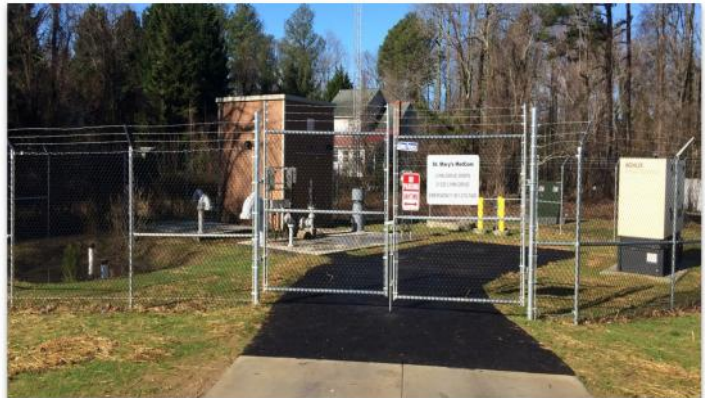
Lynn Drive WWPS & Forcemain Replacement: Station After Replacement
