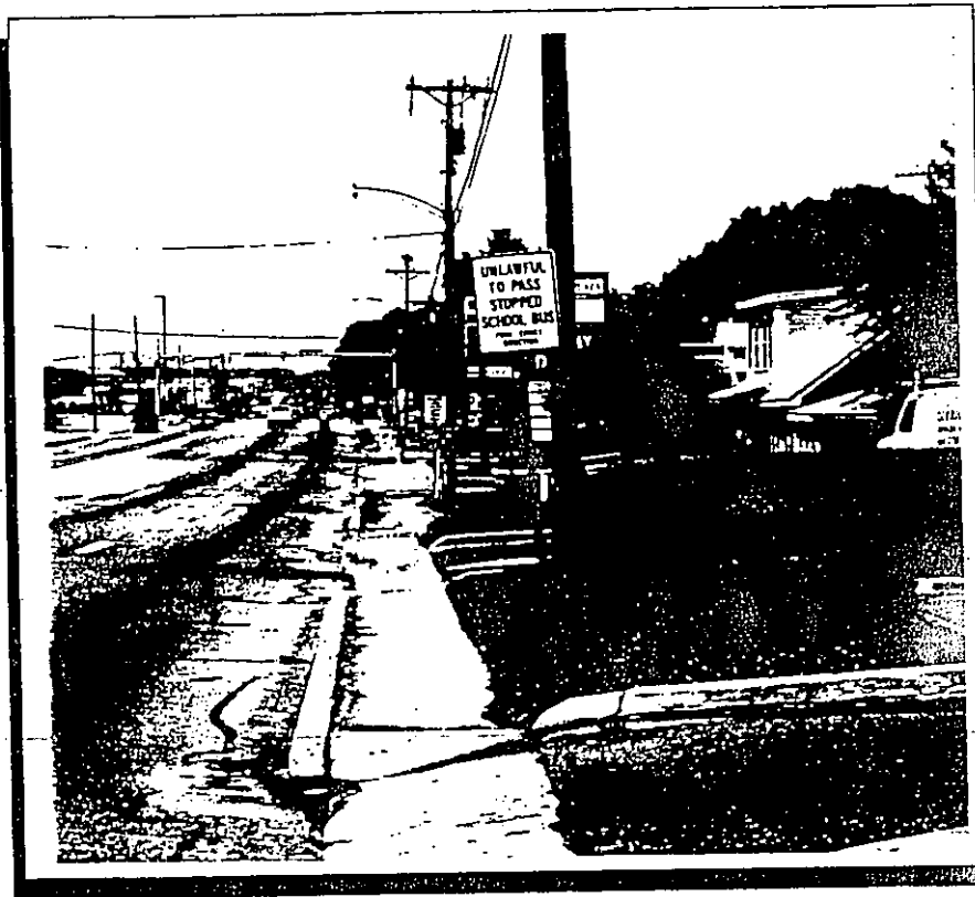
Photo 4. Great Mills Road looking west. Sidewalks in poor condition and numerous curb cuts discourage pedestrian activity.
