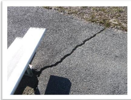
**Access issue:** Access path is damaged with cracks larger than ¼'
