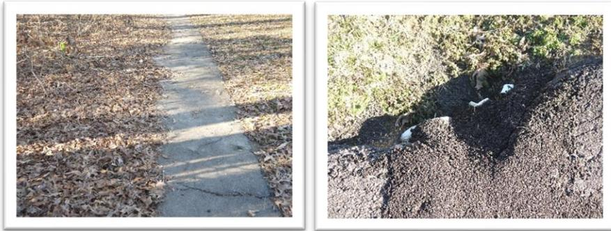
**Access issue:** Access path is damaged with cracks larger than ¼' and covered in debris
